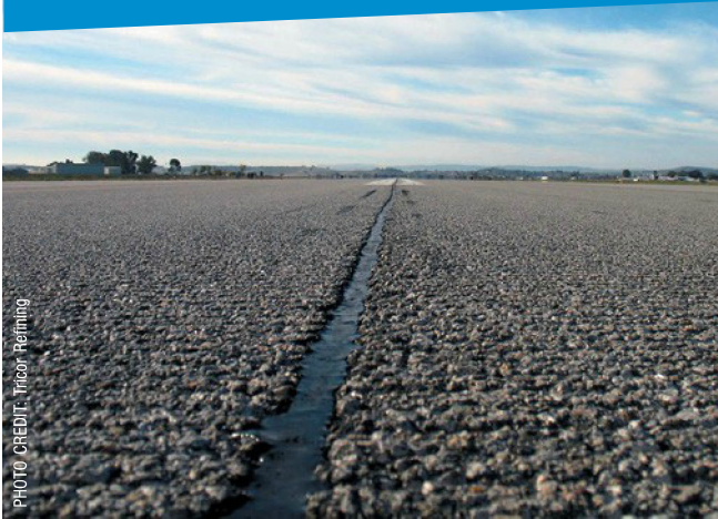
PHOTO CREDIT: Tracor Rejuvening At Paso Robles Airport, unsealed grooved asphalt was crack-sealed prior to rejuvenator application
